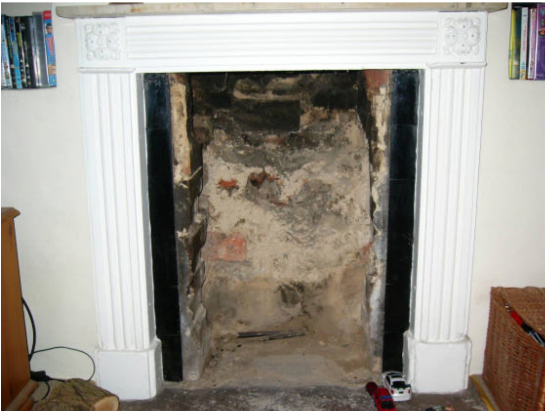
Figure 1. The original fireplace and rubble fill.
