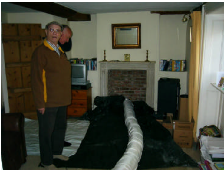
Figure 8. Liner being pulled up the chimney
