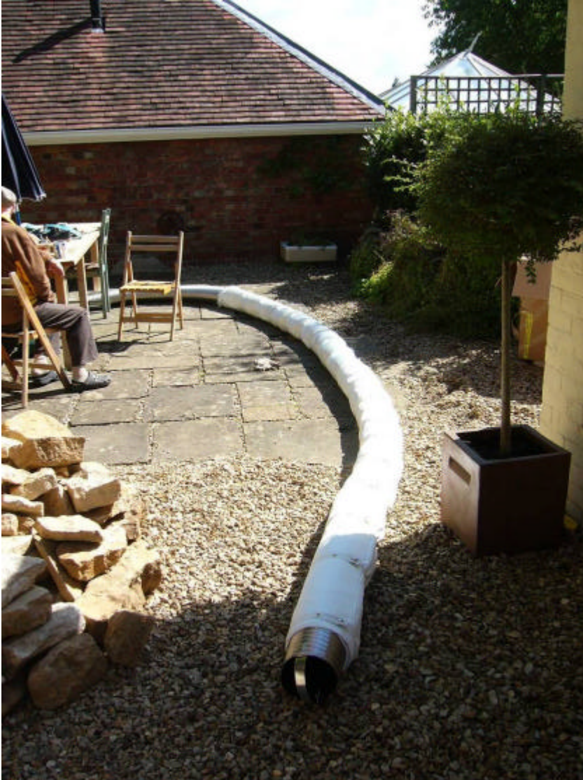
Figure 6. The flexible stainless liner and Chimwrap insulation.
