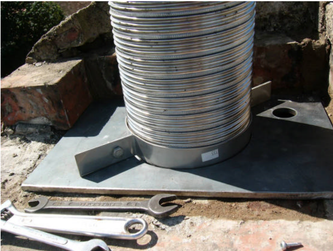
Figure 9. The top closing plate incorporating the chimney vent
